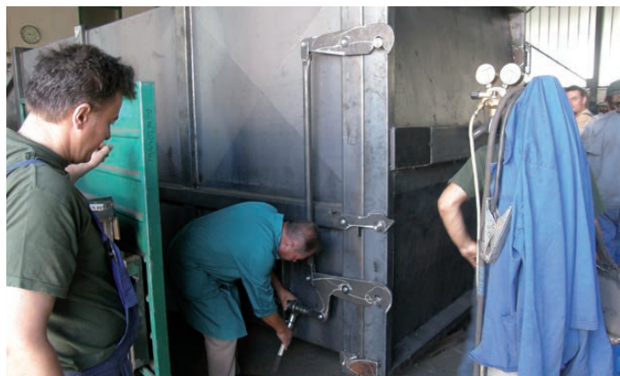
MONTAŽA MEHANIZMA ZA ZATVARANJE VRATU DOOR LOCKING MECHANISM INSTALLATION
