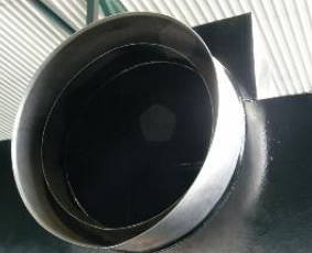
ULAZNA CIEV SEPARATORA SEPARATOR INLET PIPE
