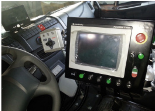
Upravljački panel - video kontrola rada sustava Control panel - video surveillance of system operation
