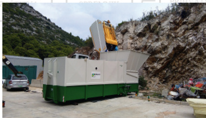
Pretovarna stanica / Transfer station
