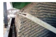
Colonies of bacteria on biological membranes of biorotor
