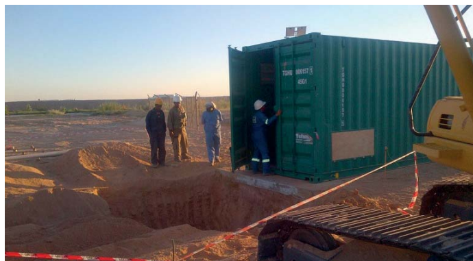
Montaža kontejnerskog Biorotora u Radničkom kampu u Iraku / Installation of biorotor container type in workers camp in Iraq
