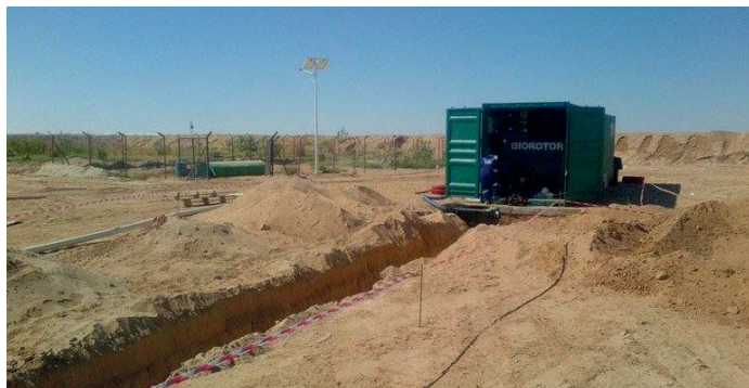
Ugradnja Biorotora kontejnerskog tipa u Iraku Construction of biorotor container type in Iraq
