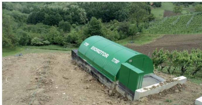
Montaža u zahtjevnim planinskim uvjetima za naselja Installation in challenging mountainous conditions for settlements
