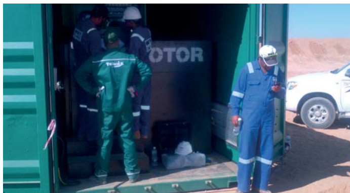
Montaža kontejnerskog Biorotora u Radničkom kampu u Iraku / Installation of biorotor container type in workers camp in Iraq
