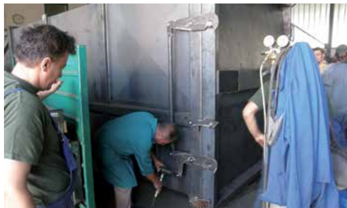
MONTAŽA MEHANIZMA ZA ZATVARANJE VRATIJU DOOR LOCKING MECHANISM INSTALLATION
